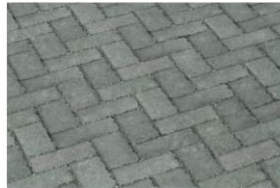
Example of permeable pre-cast concrete paving - mottled effect, laid herringbone for the service access area
